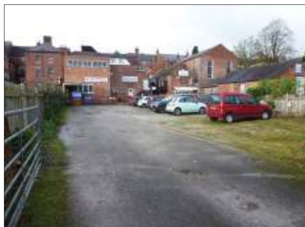
Figure 7 The Gingerbread shop of 1492 on St John's Street and a croft behind St John's Street
