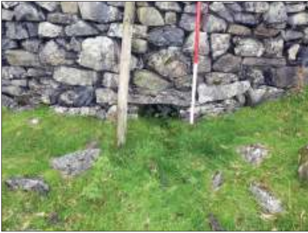
Fig. 5 Know Gap Sike with a section of glazed earthenware pipe visible
