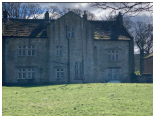
14 Mewith Head Hall, rear (north), March 2024
