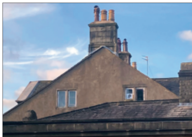
11 Detail of the south chimney of Midland Bank Chambers
