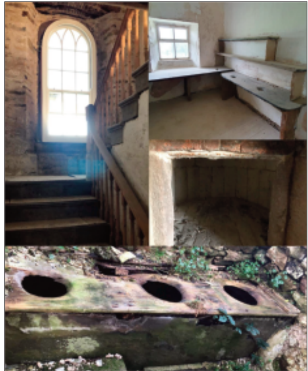
Roome Today (under renovation) :Clockwise from top left: Georgian stair and window, 17th century dairy & Georgian window, 17th century bread oven, 17-18th privy ("The Necessary")
