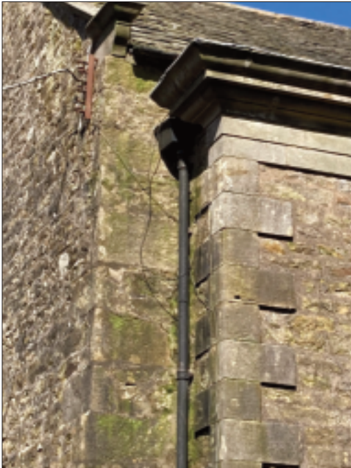
15 The south-west corner of Mewith Head Hall showing the way in which the facade does not reach the corner of the building behind.
