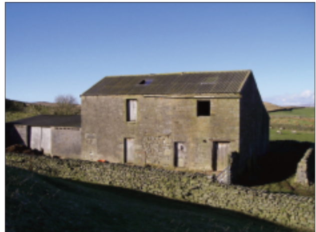
Figure 2. Bullhurst farm, now a field barn
