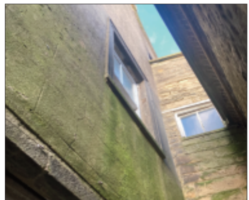
10 First floor window in south gable of Midland Bank Chambers
