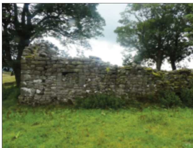
Figure 5. Unnamed farmstead south of Cockley Bank
