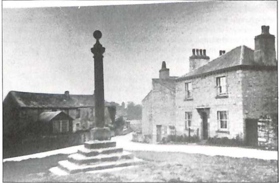
Austwick, The old Weaving Shed.
