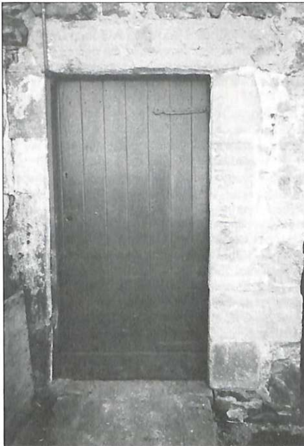
Staggarth showing old lintel (seen vertically on right of door) reused in door jamb. Photo—Maureen Ellis.
