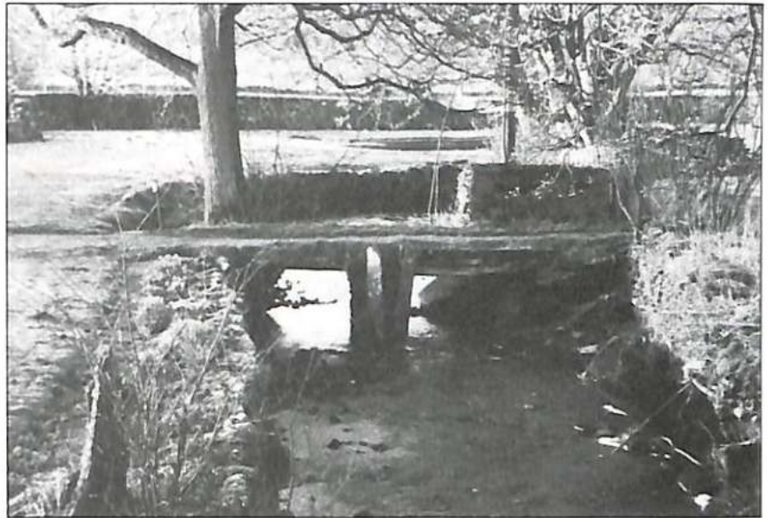
Clapper Bridge near Austwick. Photo—Maureen Ellis.
