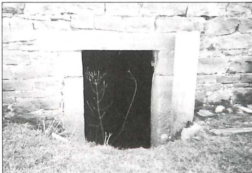
Entry to water wheel housing Runley Bridge mill.
