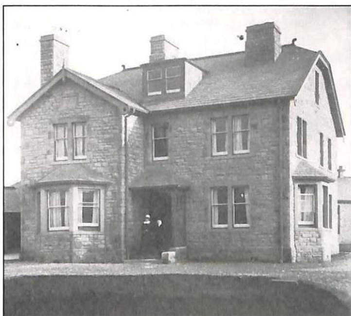
Administration Block and original front entrance. Photo by Thomas Armistead Foxcroft.
