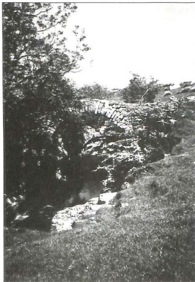
Packhorse Bridge over Gayle Beck. Photo—Maureen Ellis.
