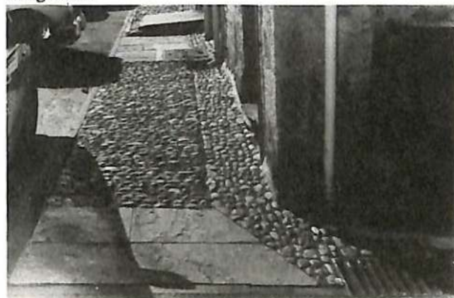
An example of the newly laid cobbles and flags.
