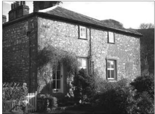
Fig. 7 The Green, south gable. The blocked first-floor door is seen on the right. (David Johnson)
