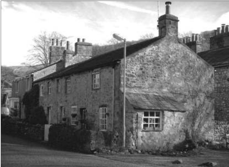
Figure 2. Left Cottages fronting Main Street. The slight change in roofline in Fountains Cottage marks the straight joint between the two original cottages. A change in quoins on the right-hand side of the near gable indicates the original steep roofline. (David Johnson)
