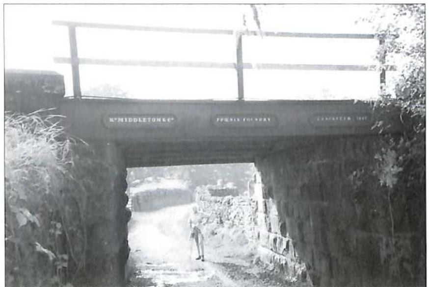
Railway Bridge made by Phoenix Foundry
